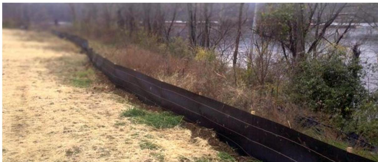
*Figure 7-13 Silt Fence Installed alongside Riverbank [Source Thrace Synthetic]*
